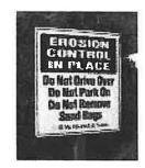
Rain that falls onto construction sites is likely to carry away soil particles and other toxic chemicals present on construction sites (oil, grease, hazardous wastes, fuel). Storm water, if not properly managed, carries these pollutants to streams, rivers, and lakes. Erosion and sediment control practices can serve as a first line of defense,
