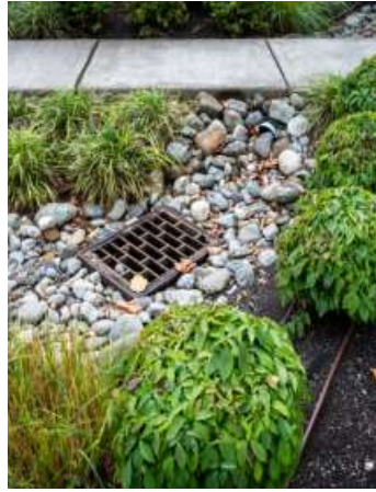
Green stormwater management example
