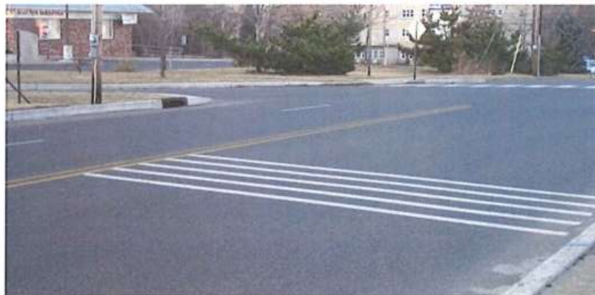
Transverse Pavement Markings
