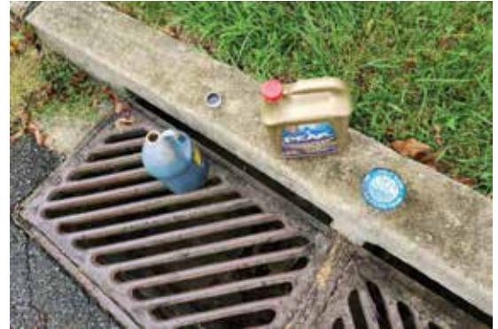
Oil and antifreeze dumped in storm sewers make their way to streams and are illicit discharges.
